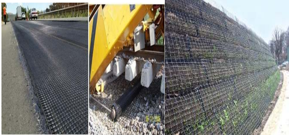
Geogrids in pavement construction and retaining wall
