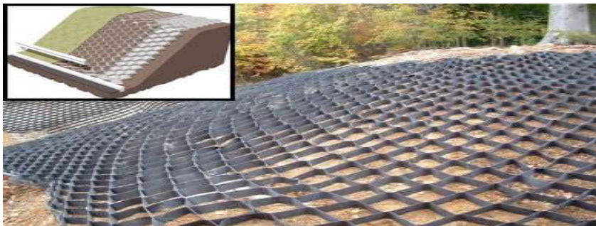
Geocells Being Filled on a Hillside Construction Erosion & Sediment Control.
