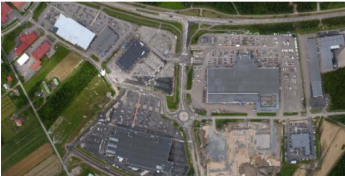
As build surveying
