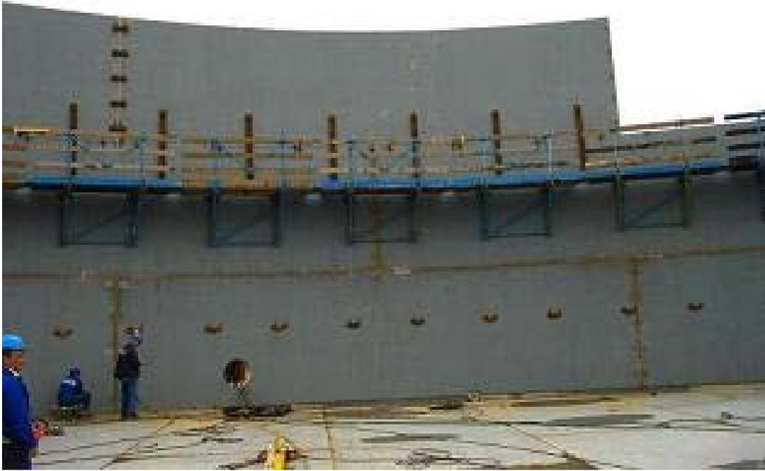
View of tank under construction and the safe scaffolding for job performing
