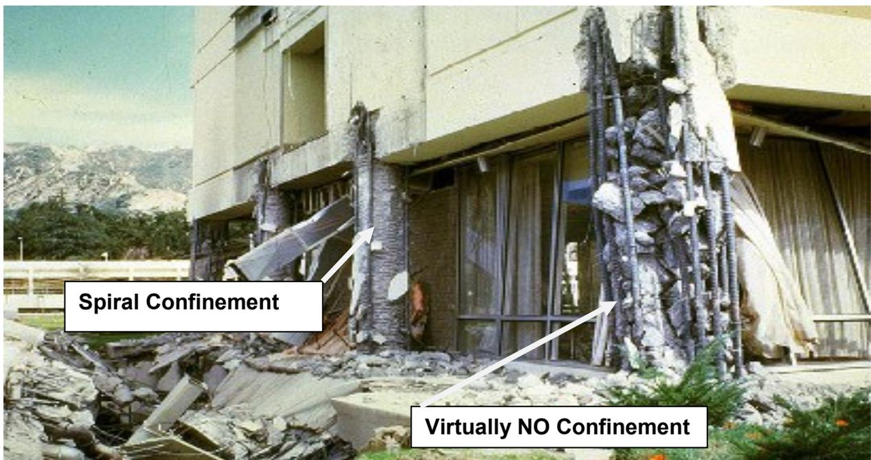
Circular spirals confine concrete far more effectively than one-dimensional ties. The helpful effects of circular spiral steel reinforcement embrace strength sweetening, a rise in strain admire most strength, and a greatly exaggerated ability of the concrete to sustain giant deformations while not vital strength loss. once concrete sections square
