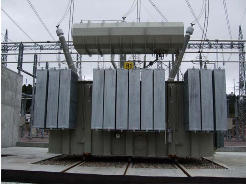
**Figure 9** Bus connected, 420 kV, 200 MVar, oil immersed shunt reactor
