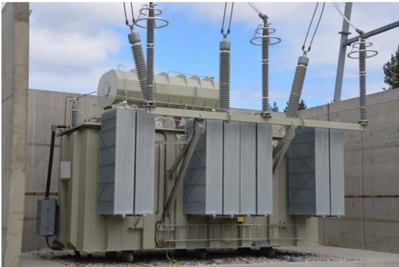
**Figure 1** Bus connected, 20.0 kV, 10.0 MVar, oil immersed shunt reactor
