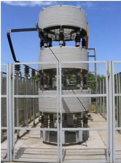
Figure 1 Aircore reactor
