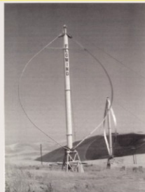
Attempts with vertical axis, 1988: Heidelberg 300kW, Flowind 170kW
