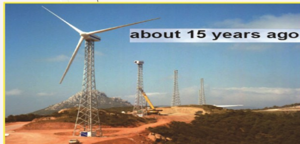
Modern Type, 1995: 600kW, horizontal axis, three blades
