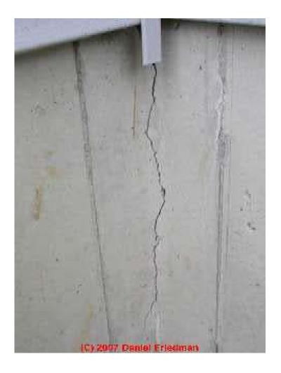
This settlement crack probably occurred during initial footing settlement. Notice that it is wider at the top than the bottom of the crack.
