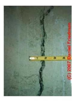
In the photos shown here, substantive cracks appeared and continued to increase in size in this poured concrete foundation used to support a modular home which had recently been completed. The cracks and foundation movement were probably due to a combination of: poorly prepared foundation footings, blasting on an adjacent building lot to prepare that site for new construction, and possibly omission of steel reinforcement in the poured wall.
