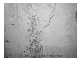
This settlement crack probably occurred during initial footing settlement. Notice that it is wider at the top than the bottom of the crack. This suggests that the footing to the left or right of the crack has moved downwards; with further downwards movement as we move further from the crack itself. If this is new construction and the crack does not change in width the site conditions may have stabilized.
